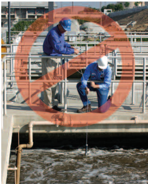
Figure 26. Photo on left shows sensor being dangled into the pond, an incorrect installation. Photo on right shows correct sensor mounting – sensor is threaded into a pipe conduit while cable is run through the pipe of the Handrail Mounting Assembly.
