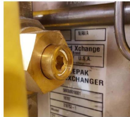
V3 INDICATOR OPEN POSITION
