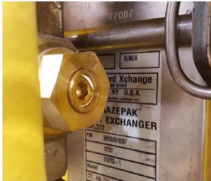
V3 INDICATOR CLOSED POSITION
