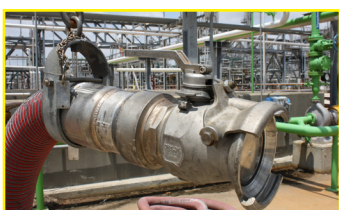
SI Group relies on OPW Drylok™ Dry Disconnect Couplers throughout its chemical plant.
